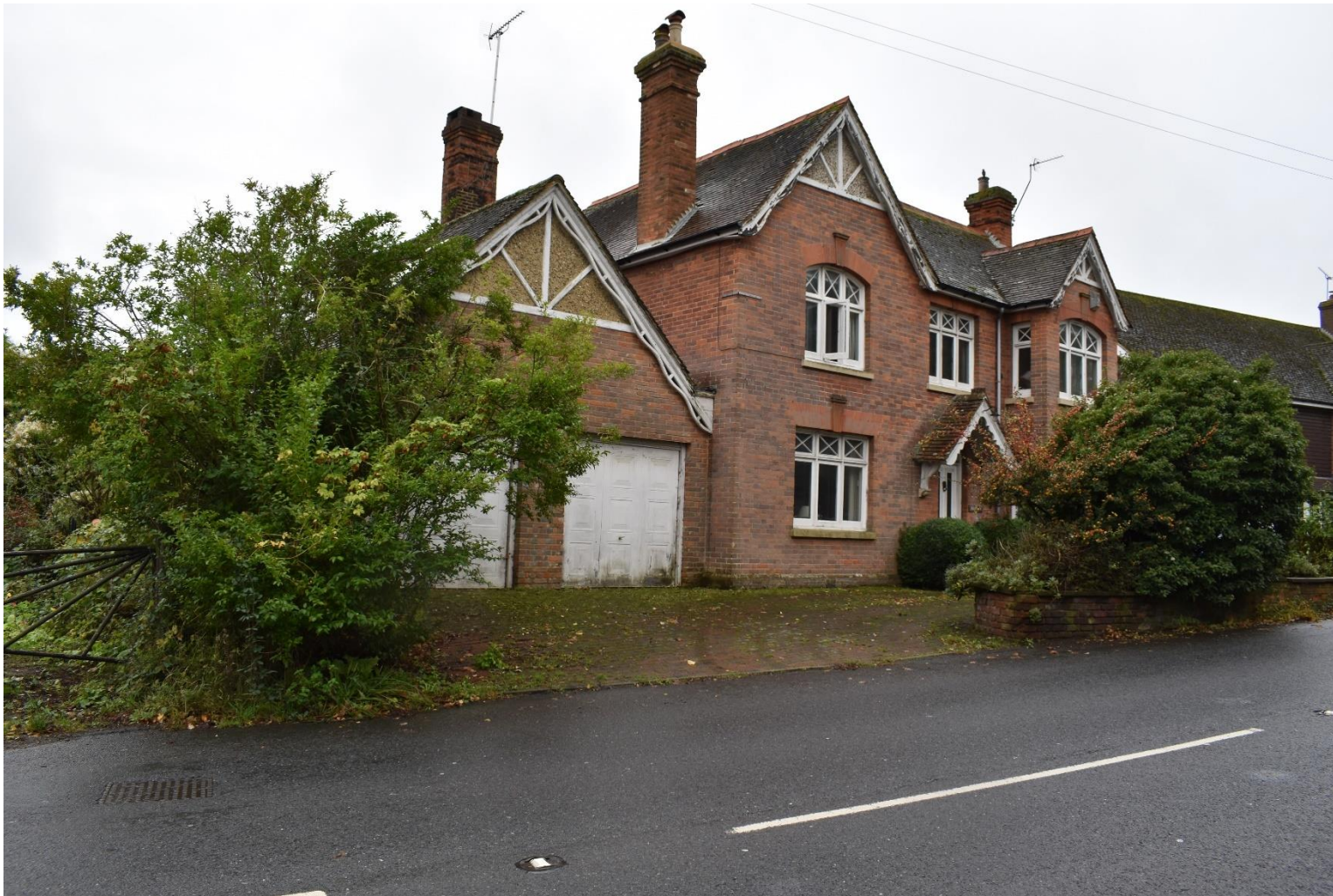
Plate 18: View of 'Bucklers' (facing WSW)
