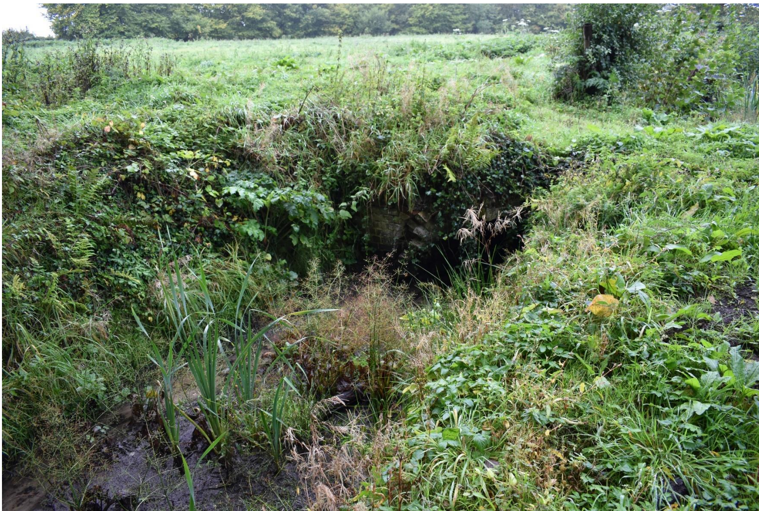
Plate 14: View of the culvert (facing W)
